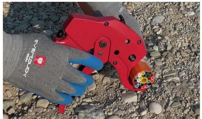
1.3 Cut end of micro duct bundle vertical and straight.
